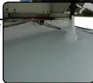
Polymeric coatings easily conform to difficult shapes and obstructions
