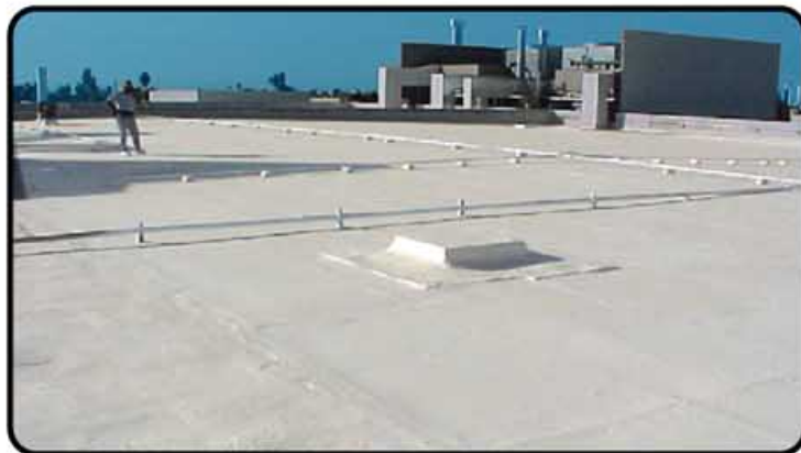
Finally, a roof that can last outlast the building it protecting
