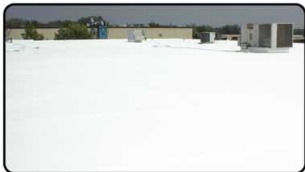
Re-surfacing of single-ply, metal roofs and built up
