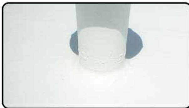
Warranted maintenance on flashings, seams and ducts
