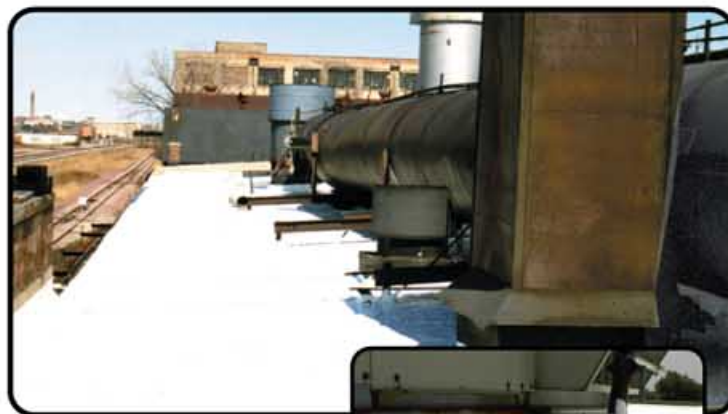
Polymeric coatings easily conform to difficult shapes and obstructions
